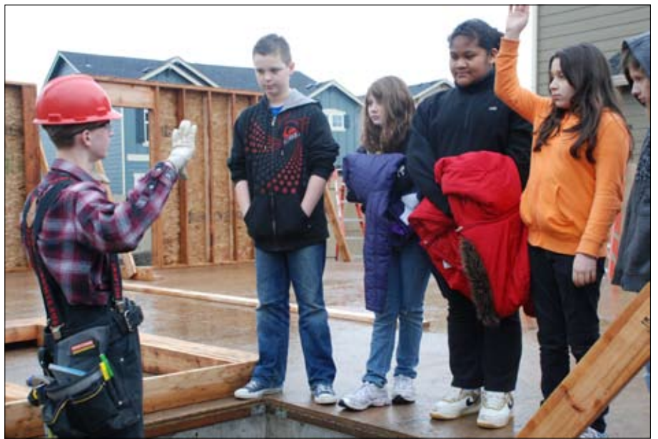
On-Site Learning: Skills Center student Carson Dodge answers questions from Endeavour Elementary School students when they visit the building site where Skills Center students are constructing a house.
